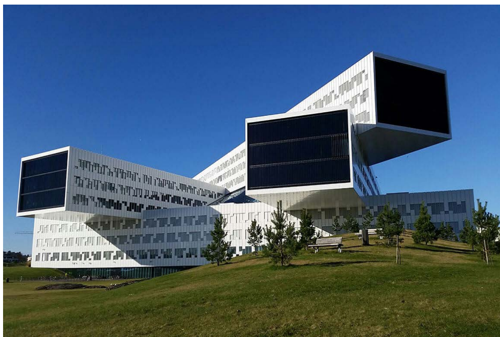
Rysunek 8. Siedziba Statoil Regional and International Offices w Fornebu pod Oslo, 2012 (Figure 8. Seat of Statoil Regional and International Offices in Fornebu near Oslo, 2012)
